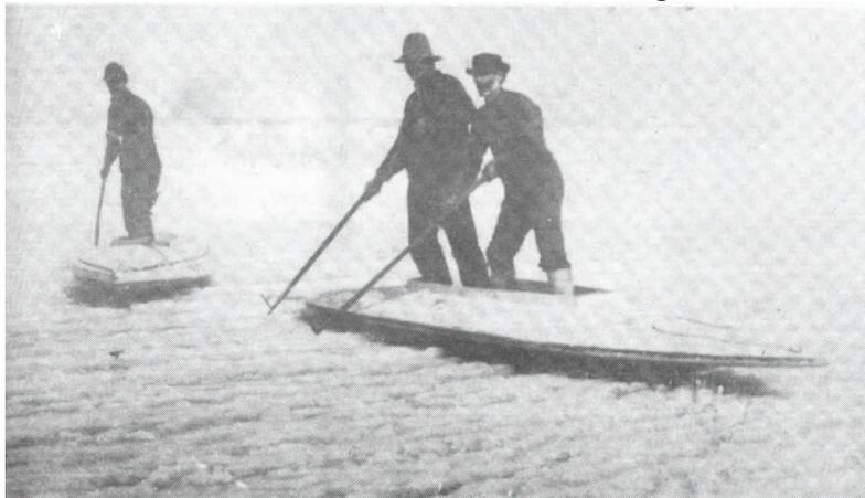
and add runners. A mast, sprit sail or gaff and a pike pole to steer her. Angle the runners (bevel) to bite into the ice and to prevent the boat from sliding sideways. Add a jib to balance the main sail and
